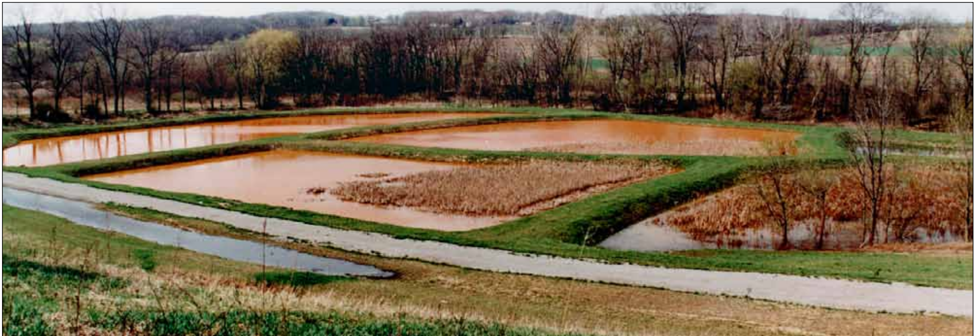
Saint Vincent passive treatment system near Latrobe
