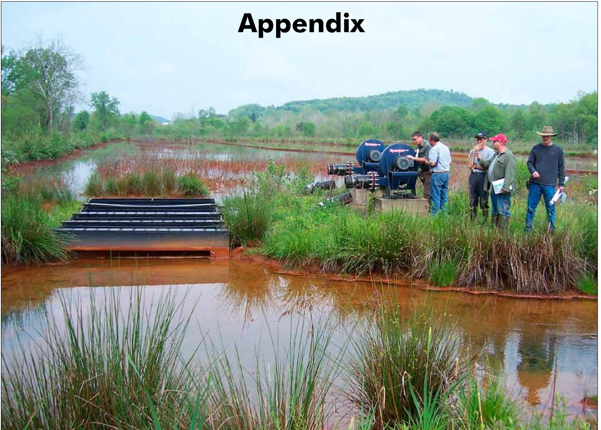
Brinkerton Treatment System, Westmoreland County
