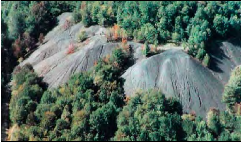
Nemaquin abandoned refuse pile
